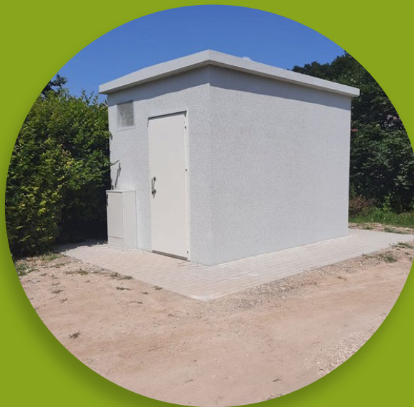
Shelters PoP fibra óptica
