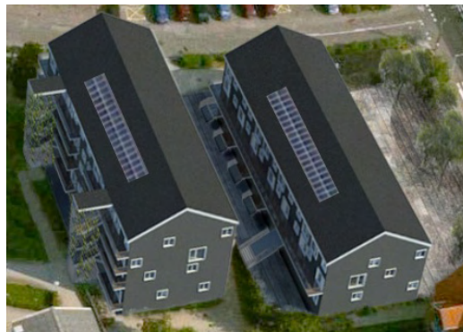
Figure 6: Sems Have, an example of renovation to NZEB.
