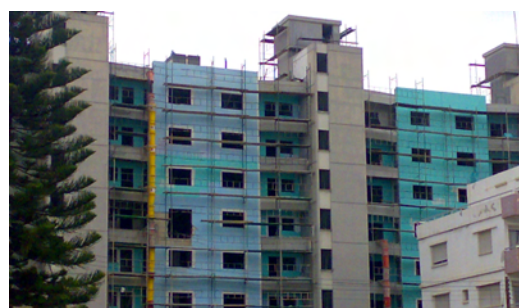
Figure 5: Renovating and upgrading the energy efficiency of an existing apartment building.
