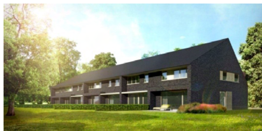
Figure 15: The 'Sustainable Quarter', NZEB houses in Waregem, with focus on affordability.
