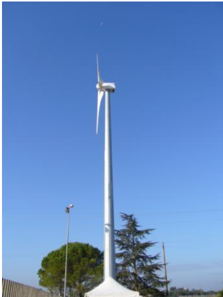
G- Turbina eólica 20 kW full-converter
